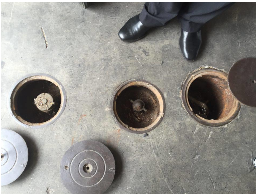
Photograph 2 – Fill and dipping points for the single UST identified.
